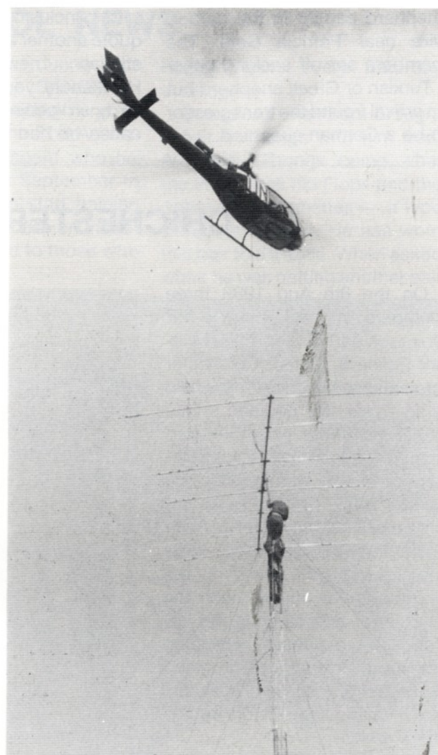
Fixing the antenna to the mast.
