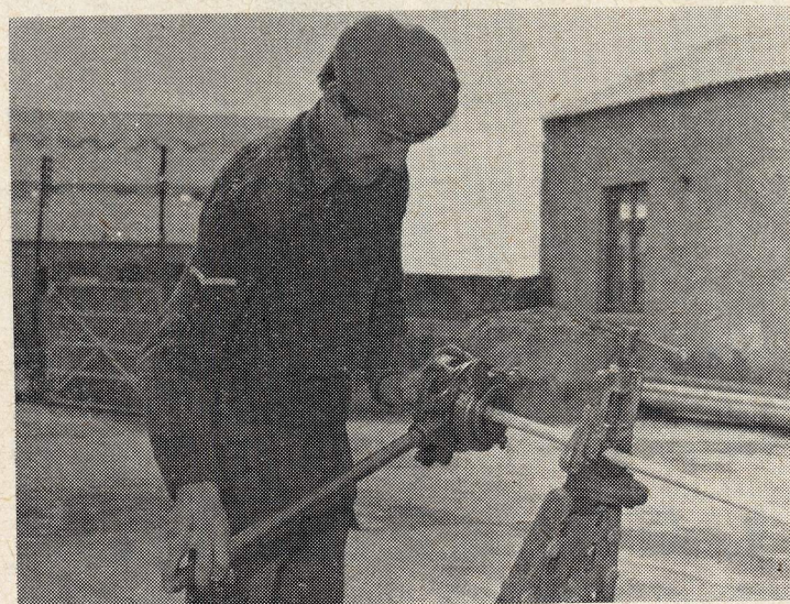
Lance Corporal G. Smith, Plumber, tapping a pipe in the RE yard at Camp UNFICYP.
