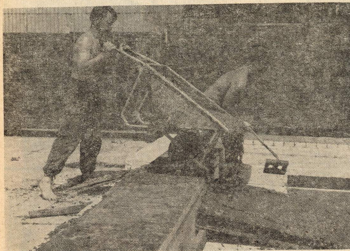
● These well dressed Engineers are repairing the Chimo Pool prior to the opening. Note the rigid position of Attention Corporal Jackson displays whilst emptying the wheelbarrow and the perfect At Ease of Corporal Pfeifer raking the concrete.
